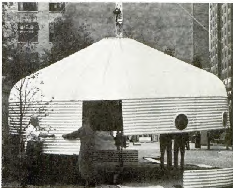
Another view of the circular metal house showing the roof being lifted on the steel mast and some of the wall sections bolted in position
